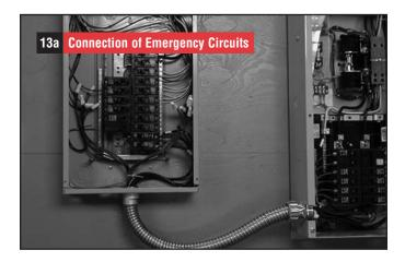
13a. Remove the main electrical distribution panel cover. Remove appropriate size knockout from the bottom or side of the main panel. (A 2-foot flexible conduit is pre-wired from the transfer switch with built-in load center.) Remove threaded lock nut from conduit coupling. Feed all wires through knockout into main panel. Slip lock nut over wires and tighten securely onto conduit coupling.
